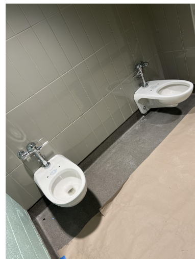
Installing plumbing fixtures in restrooms on level 2
