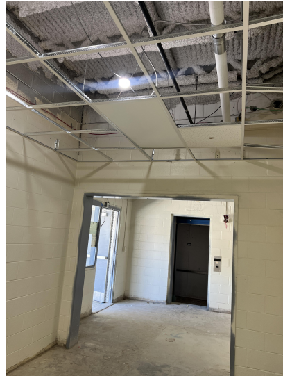
Installing ceiling grid and painting in corridor on level 1.
