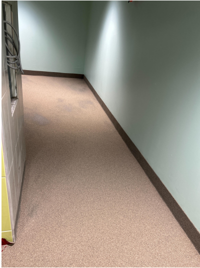
Installing resinous flooring on level 2.
